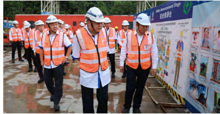
董事长王彤宙在马来西亚开展项目安全检查 Chairman Wang Tongzhou carried out project safety inspection in Malaysia
