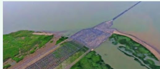
长江南京以下 12.5 米深水航道一期生态环保项目 Ecological and Environmental Protection Project of Phase I of 12.5m Deep Water Channel below Nanjing on the Yangtze River
