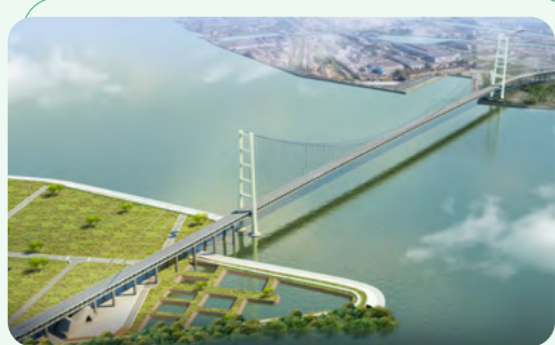
Shiziyang Corridor Engineering
