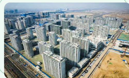
雄安中交未来科创城综合开发项目 Xiong'an CCCC Future Science and Technology Innovation City Comprehensive Development Project
